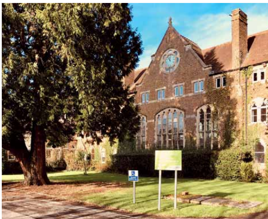
The former Adult Education Centre in Sittingbourne – one of Swale’s many listed buildings
