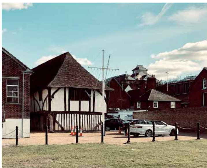
The TS Hazard building, Faversham.
